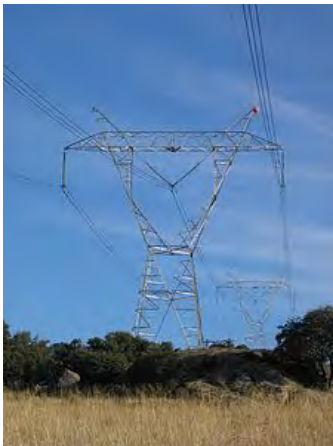
Overhead high-voltage power lines
