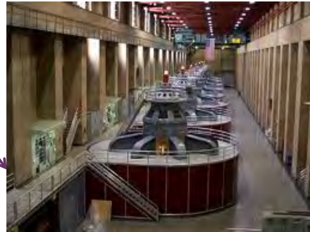
Large AC generators at Hoover Dam.
