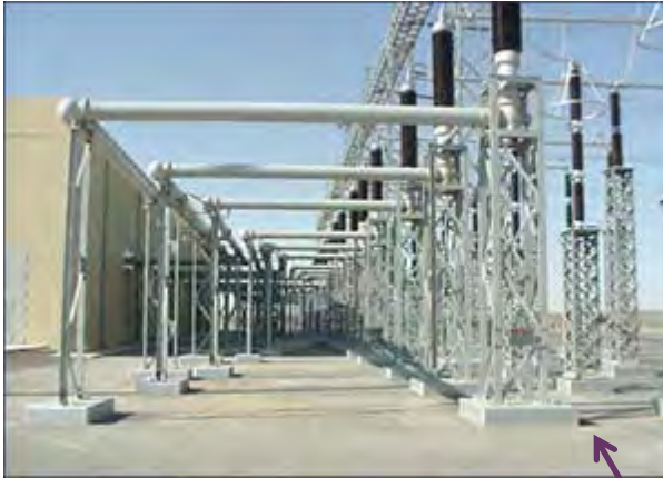
Power buses in a substation.
