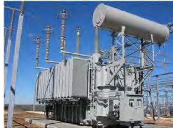
A transformer in a substation.
