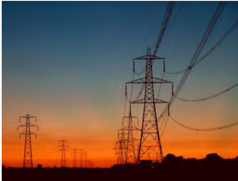
Power transmission and distribution.
